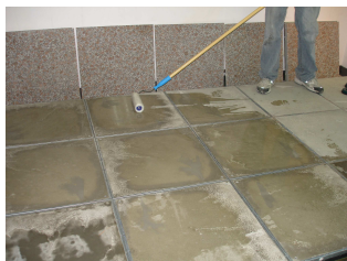
rinse panels and tiles
