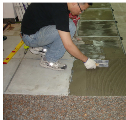
apply adhesive on panels
