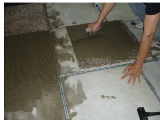
apply adhesives on tiles
